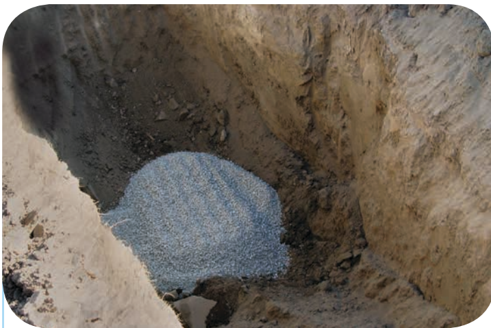
Example of a bentonite topseal installed during the decommissioning of bored well
